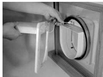
When fitting the Petporte smart flap into an opening offer the interior section with Extension Tunnel if needed up to the opening. Next pass the porch cable from the porch and exterior section through the rectangular opening in the interior section.
